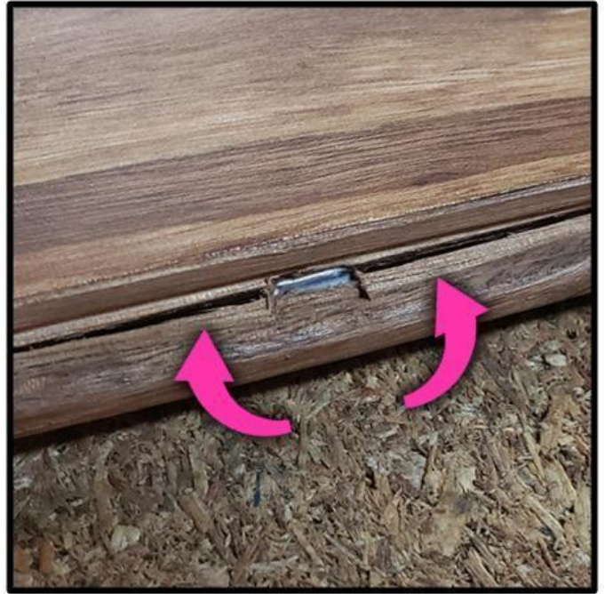
Cleat properly driven and some splitting
