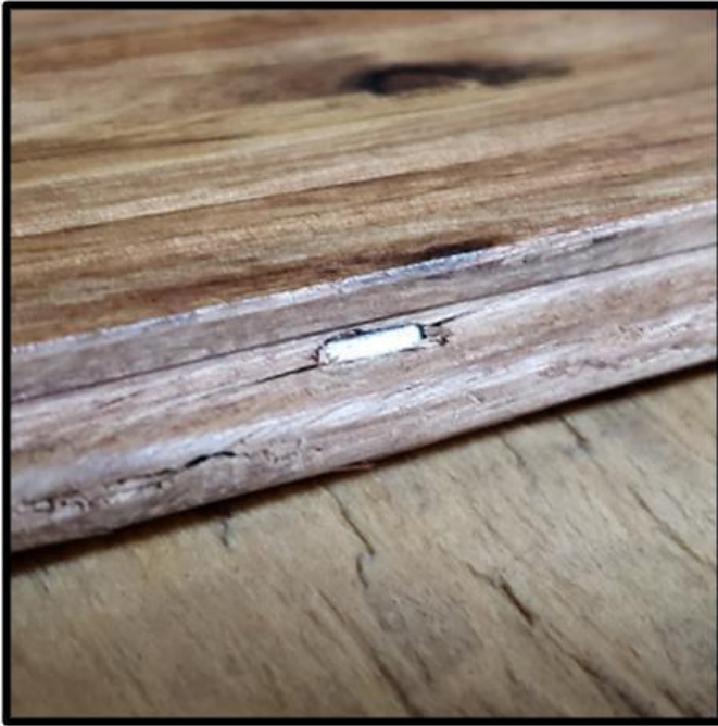
Cleat properly driven and no splitting
